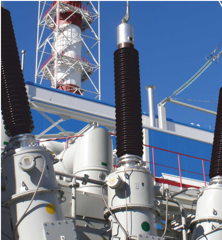
220 kV bushings in a transformer at HPP
